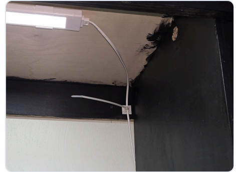
Tie threaded and pulled snug.
